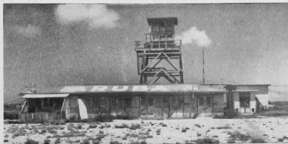
No, it isn't a toolshed or a chicken coop, it's the old airport building, Aruba's first air-link with the outside.
